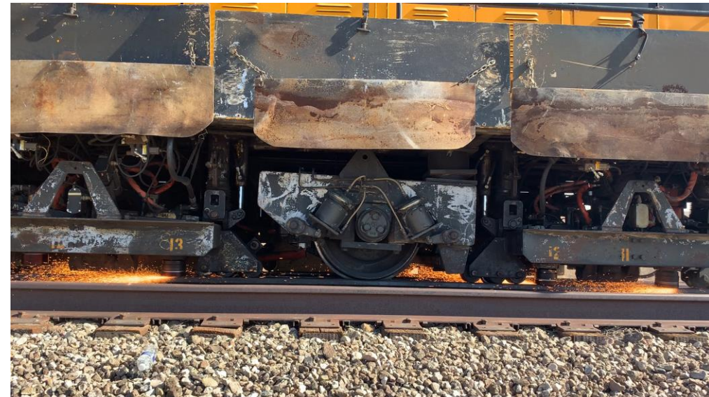
Rail Grinding Operation
